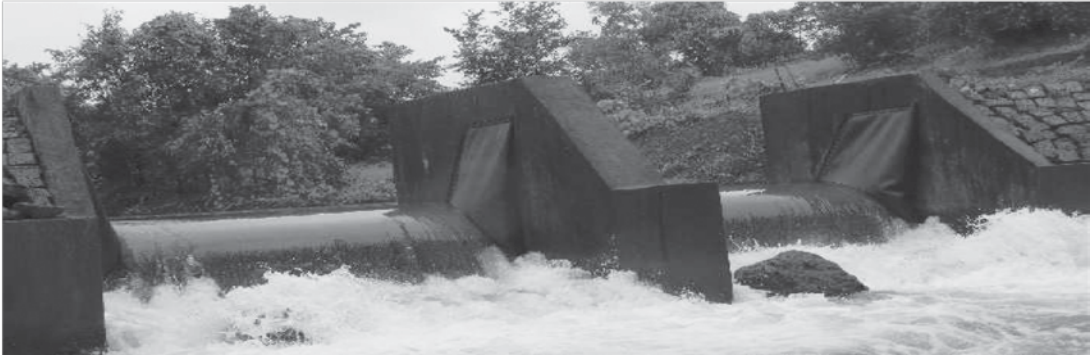
Plate 1. Rubber dam at Konkan region, Dapoli
