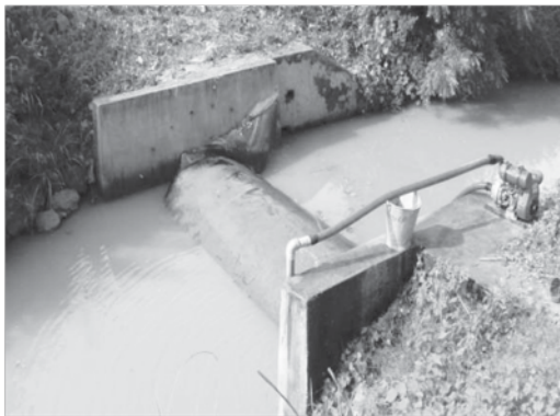
Plate 2. Rubber dams installed in watersheds of Odisha by IIWM, Bhubaneswar
